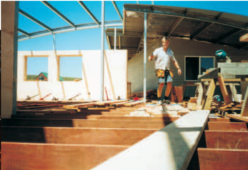
Gary building the family home in Margaret River.
